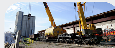
SPECIAL AND PROJECT TRANSPORTS
